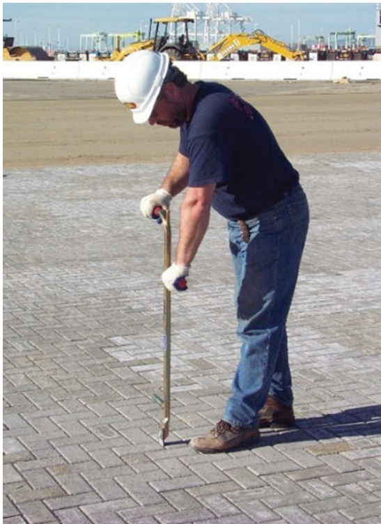
Figure 41. An alignment bar and string line can be useful to tweak the pattern and make it line up with the surrounding undisturbed paver.
