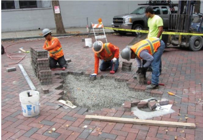
Figure 40. Pavers salvaged during the disassembly can be brought back and placed according to the original pattern. Care needs to be taken to ensure any remaining sand on the bottom or sides of the pavers is removed before placement.
