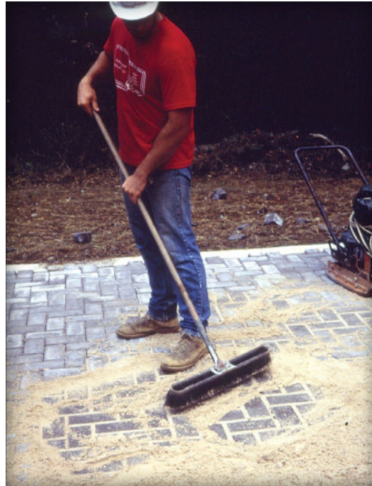
Figure 10. Spreading the joint sand.
