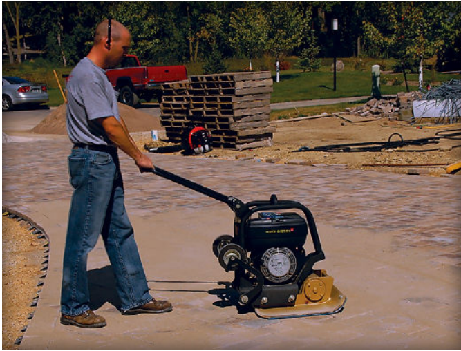
Figure 11. Vibrating sand into the joints.
