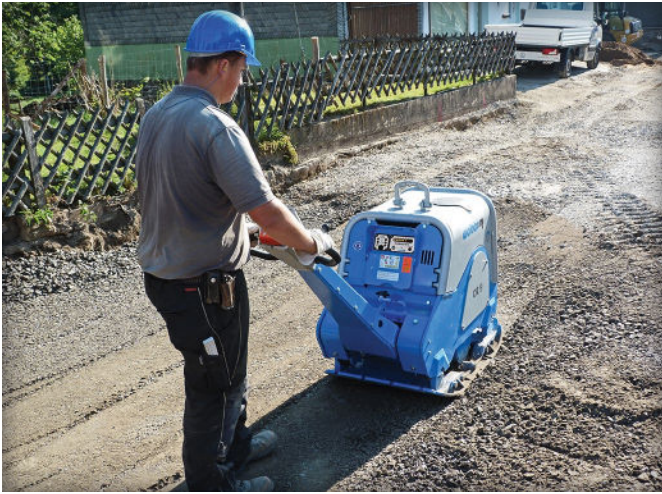
Figure 4. Base compaction with a reversible plate compactor.
