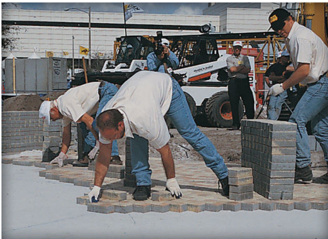
Figure 7. Placing the concrete pavers.
