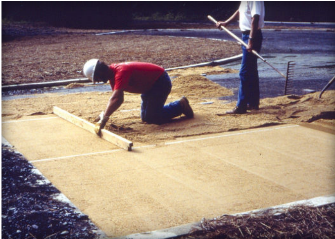
Figure 6a & 6b. Screeding the bedding sand.
