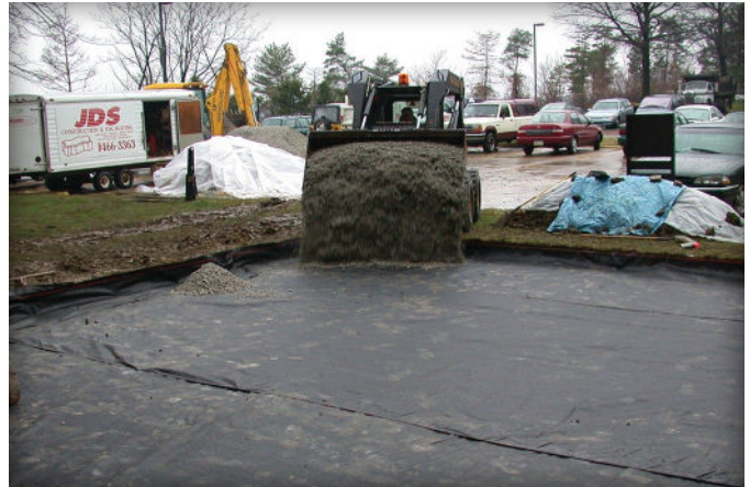
Figure 3. Application of the geotextile under aggregate base.
