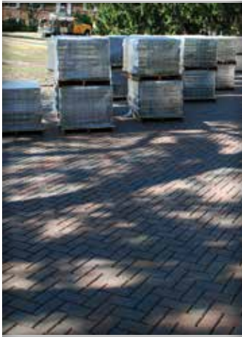
Figure 2. Bundles of ready-to-install pavers for setting by mechanical equipment. Bundles are often called cubes of pavers.
