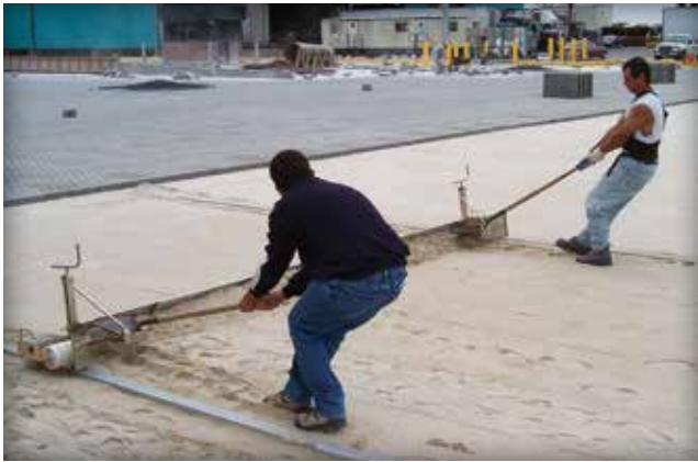
Figure 4. A two-man hand pulled screed
