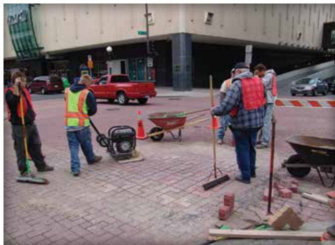
Figure 15 and 16. Reinstated pavers leave no ugly patches nor do they weaken the pavement.
