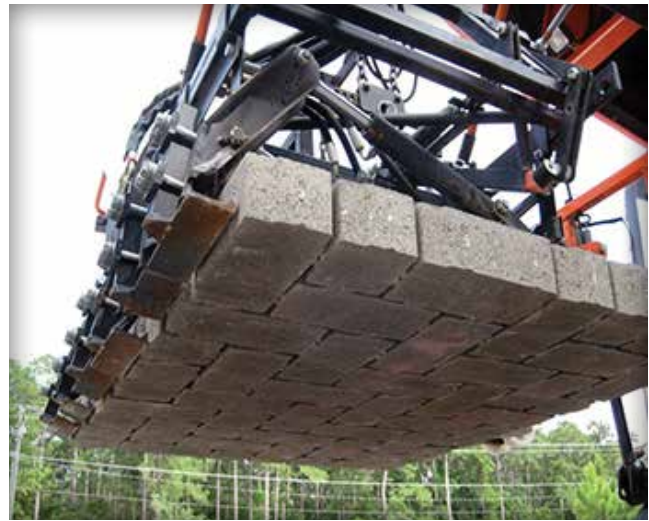
Figure 3. A cluster of pavers (or layer) is grabbed for placement by mechanical installation equipment. The pavers within the cluster are arranged in the final laying pattern as shown under the equipment.
