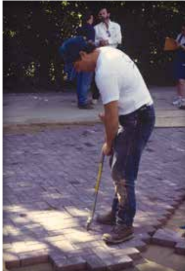
Figure 13 (Left). Adjusting joint spacing and alignment. Figure 14 (Right). Second and final compaction of the pavers. The first compaction occurs after the pavers are placed (no sand in the joints). The second compaction works the sand on pavers into the joints. This process causes the pavers to interlock.
