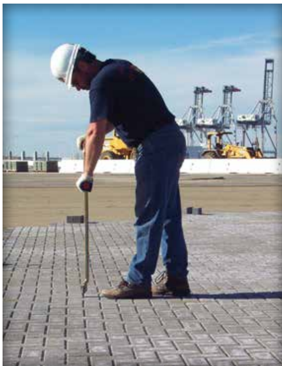
Figure 20. Adjusting joint lines with a pry bar prior to compaction.
