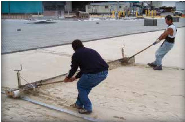
Figure 4. A two-man hand pulled screed
