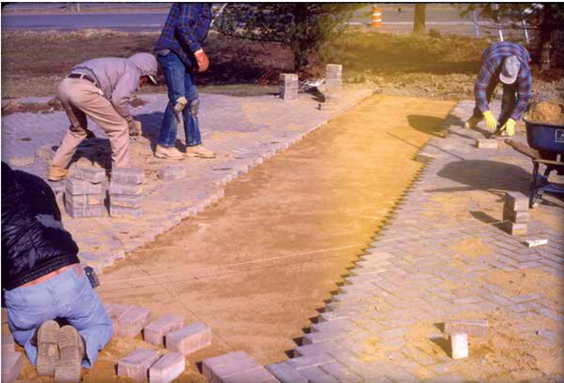
Figure 12. Screeded bedding sand. Note that a few courses of pavers are removed to create even sides for screeding. Installing temporary edge restraints prior to excavating is preferred practice.
