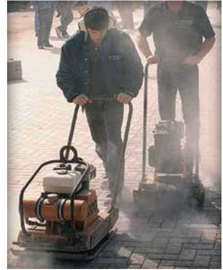
Figure 13 (Left). Adjusting joint spacing and alignment. Figure 14 (Right). Second and final compaction of the pavers. The first compaction occurs after the pavers are placed (no sand in the joints). The second compaction works the sand on pavers into the joints. This process causes the pavers to interlock.
