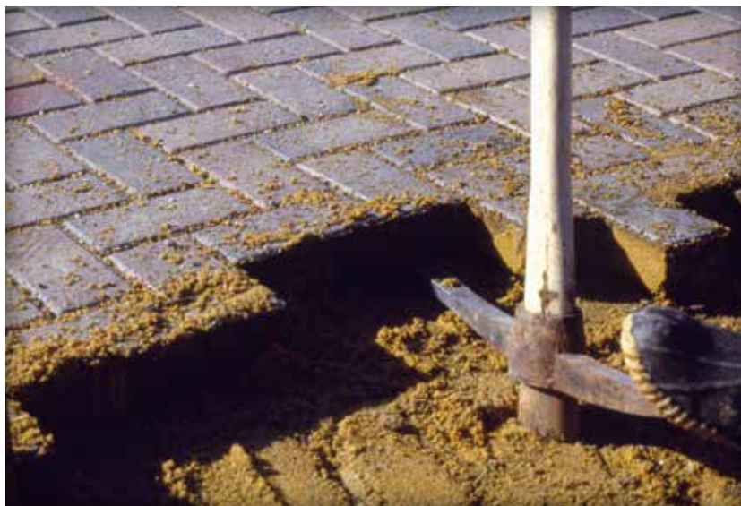
Figure 6. Prying out the remaining pavers
