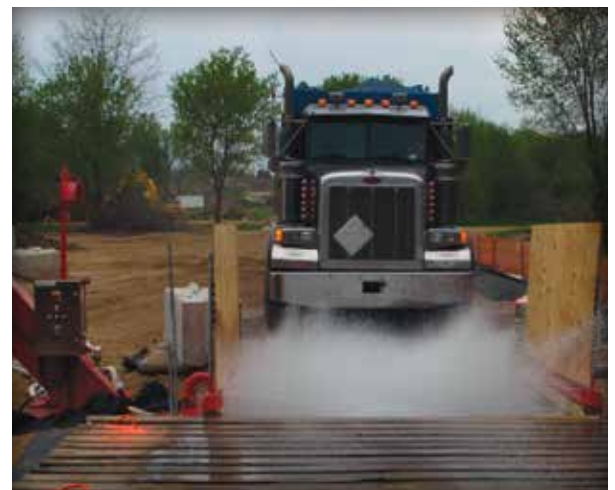
Figure 4-3. Larger PICP projects may require tire washing equipment for trucks to keep mud from contaminating PICP aggregates.
