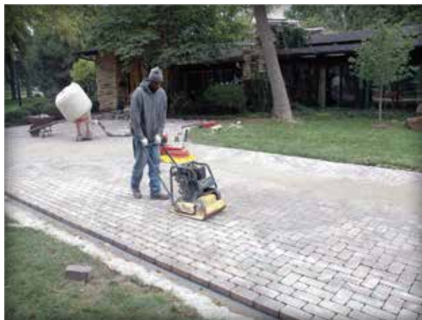
Figure 4-18. Plastic edge restraint is spiked into the dense-graded base berms so it can hold the pavers in place during compaction and service.
