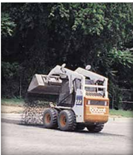
Figure 4-30. Various methods of filling and sweeping PICP joints.
