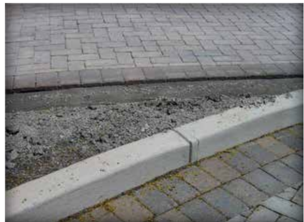
Figure 4-19. A PICP walk with a troweled concrete toe sits next to a driveway with a formed and cast-in-place concrete curb. Concrete toes should only be used for pedestrian applications.
