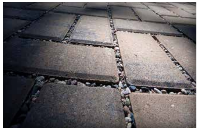
Figure 5-3. Keeping PICP joints filled with permeable aggregate facilitates removal of accumulated sediment.
