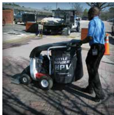
Figure 5-17. Walk-behind vacuum cleans a small parking area. Use a screen over the intake to prevent jointing stone ingestion.
