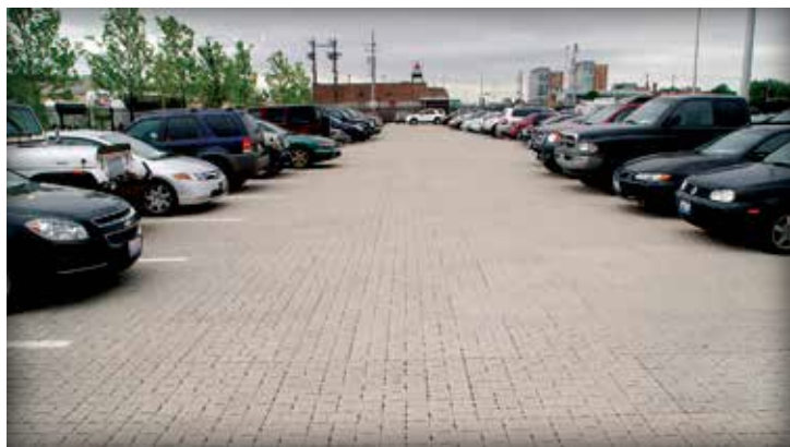
Figure 2-16. Maxwell Street Market Plaza winter temperature monitoring by the City of Chicago demonstrated the insulating effect of the aggregate. This condition precluded heaving.
