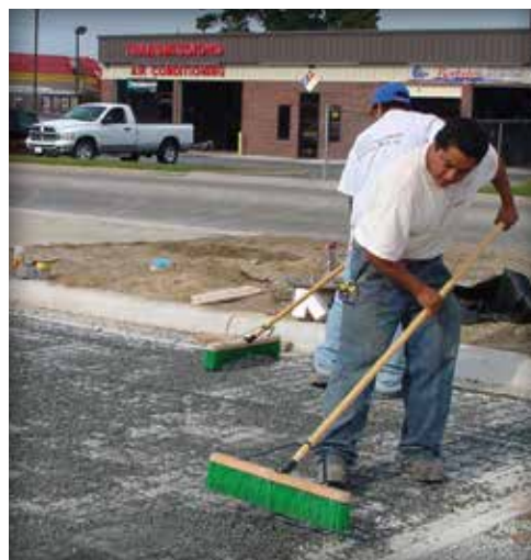
Figure 4-30. Various methods of filling and sweeping PICP joints.
