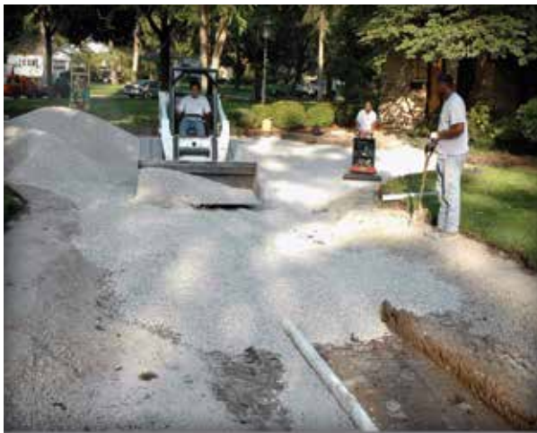
Figure 4-16. Perimeter berms made with dense-graded base are in place prior to placing open-graded aggregate in the driveway.
