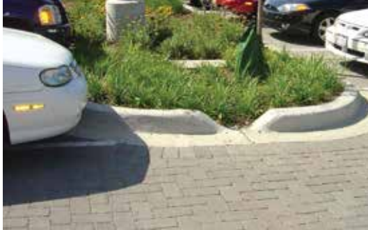
Figure 2-4. Elmhurst College, Elmhurst, Illinois, parking lots use full infiltration through the soil subgrade with overflows directed through curb inlets into bio-retention areas and overflow drains to manage extreme rain events.
