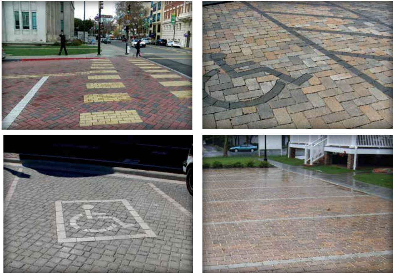
Figure 2-15. Various examples of pavement markings using PICP.
