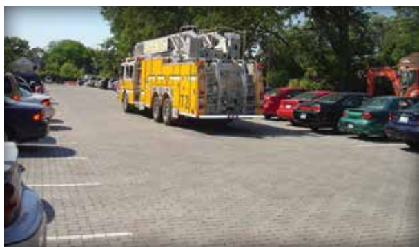
Figure 1-7. Elmhurst College, Elmhurst, Illinois, uses PICP parking lots for runoff control and water harvesting.
