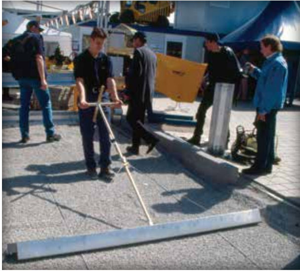
Figure 4-24. A hand screed is used for screeding the bedding layer in small areas.
