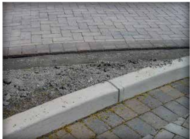
Figure 4-19. A PICP walk with a troweled concrete toe sits next to a driveway with a formed and cast-in-place concrete curb. Concrete toes should only be used for pedestrian applications.
