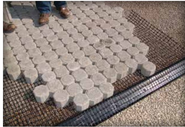
Figure 4-23. Geogrid is wrapped around this plastic edge restraint.
