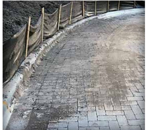
Figure 5-2. Whether eroded onto or dumped on PICP, erosion and sediment control are essential during construction.
