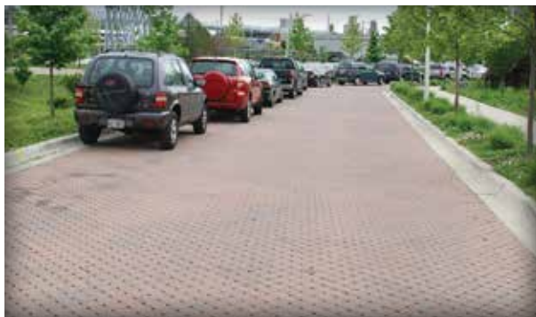
Figure 1-5. Ferdinand Street in Chicago is paved with PICP as part of a city redevelopment project.
