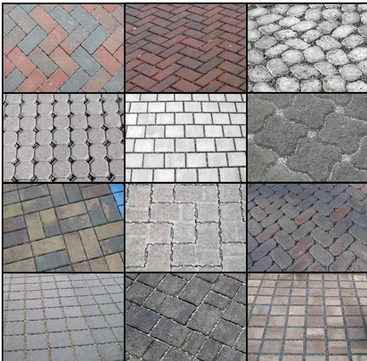
Figure 1-3. Various types of paving units used in PICP
