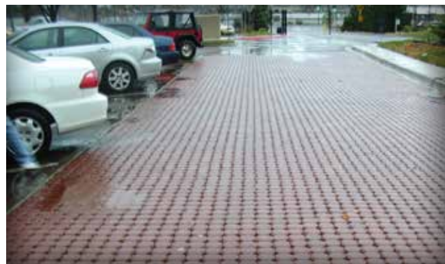
Figure 5-10. Ponding on PICP typically first occurs at the junction with impermeable pavement.
