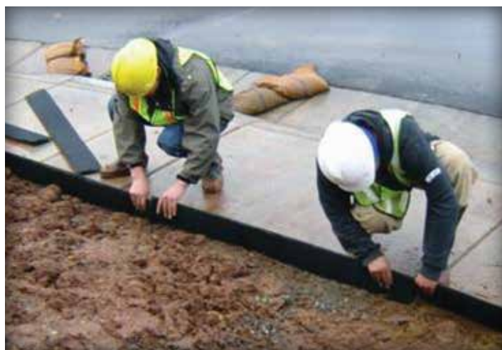
Figure 4-2. This temporary permeable edging around bare soil replaces silt fencing because it restrains sediment while allowing water to pass.
