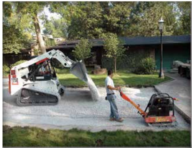
Figure 4-17. Compacting the berms along the perimeter and the PICP base.
