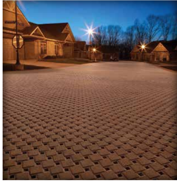
Figure 1-10. Autumn Trails in Moline, Illinois used 39,000 sf (3,900 m 2 ) of PICP without storm sewers, making it cost-competitive with conventional paving with drainage.
