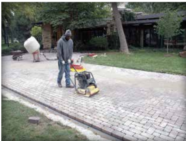
Figure 4-18. Plastic edge restraint is spiked into the dense-graded base berms so it can hold the pavers in place during compaction and service.
