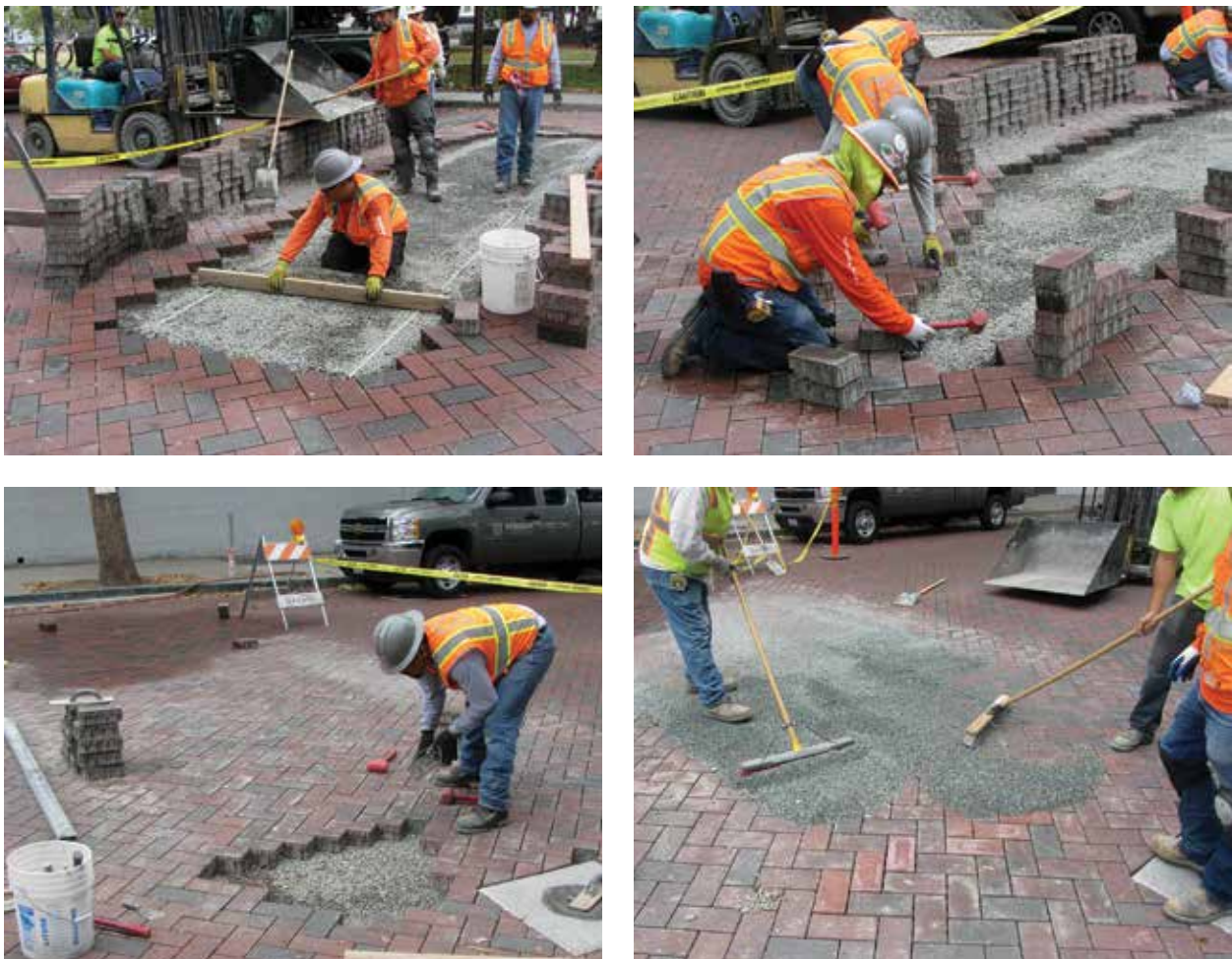
Figure 5-24. Reinstatement of concrete pavers in a PICP street.
