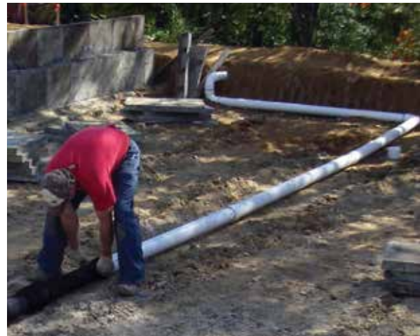
Figure 2-7. A non-perforated, raised outlet pipe is another way to achieve detention and partial infiltration. The pipe positioned on the soil is perforated.
