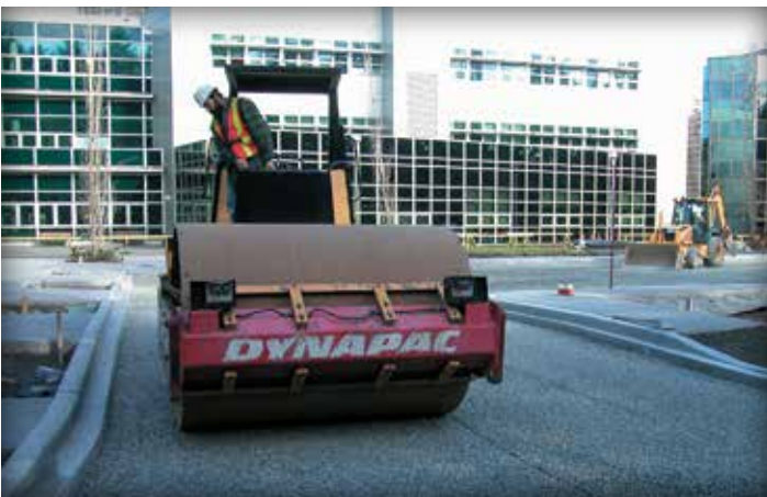
Figure 4-8. A 10 ton (9 T) roller compacts the ASTM No. 57 base.
