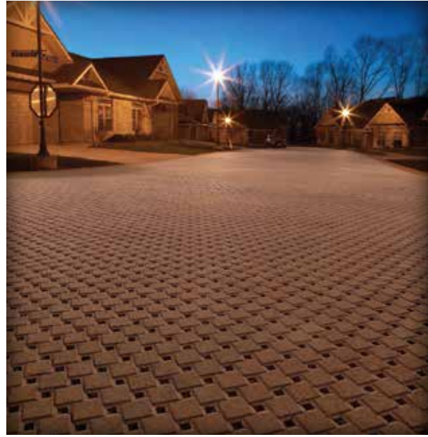
Figure 1-10. Autumn Trails in Moline, Illinois used 39,000 sf (3,900 m 2 ) of PICP without storm sewers, making it cost-competitive with conventional paving with drainage.
