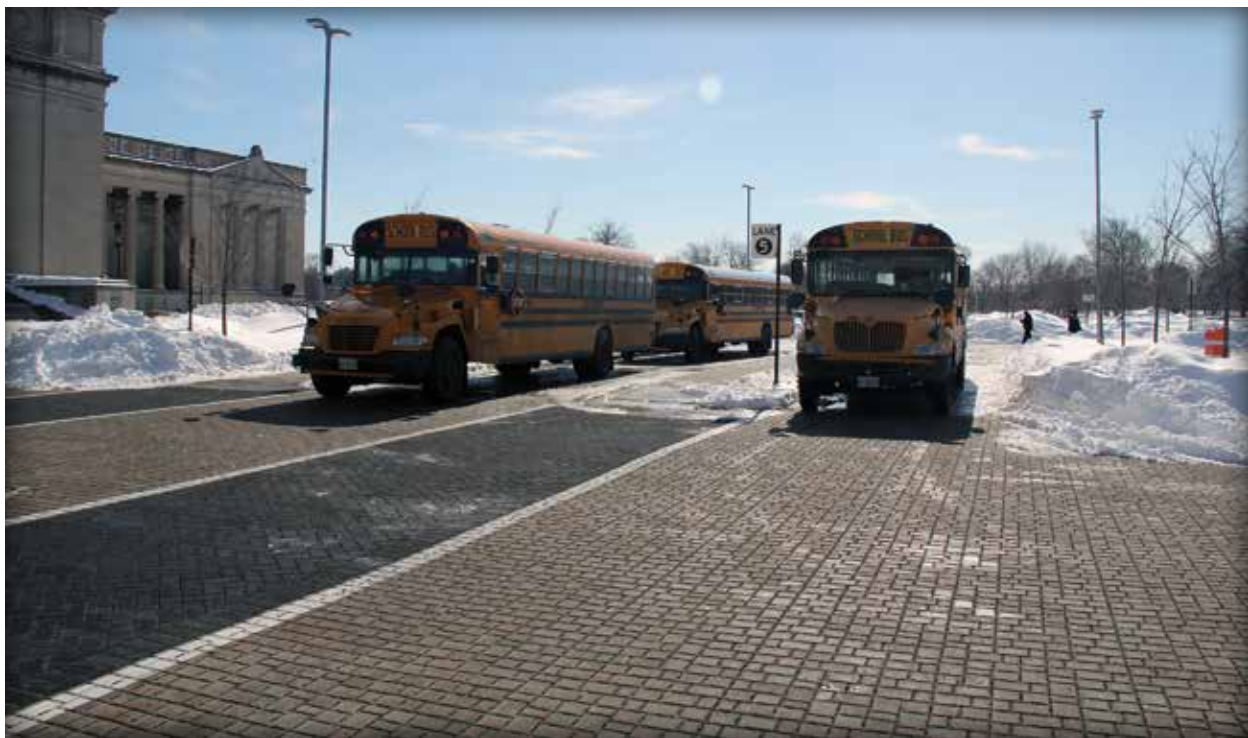
Figure 2-17. Upon plowing with standard plowing equipment, remaining snow can melt with water immediately entering the PICP surface. This reduces deicing and sand materials use as well as reducing liability hazards from slipping on ice.
