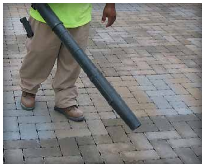
Figure 5-14. Blowing debris to curbs or gutters for removal and disposal.
