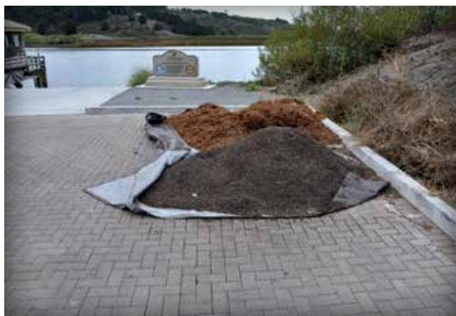
Figure 5-4. Mulch placed on tarps prevents more expensive cleaning of PICP.
