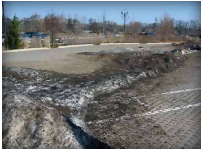
Figure 5-23. This is an example of snow that should have been deposited on a grassy area. If such areas are not available, then vacuum clean the PICP in the early spring.
