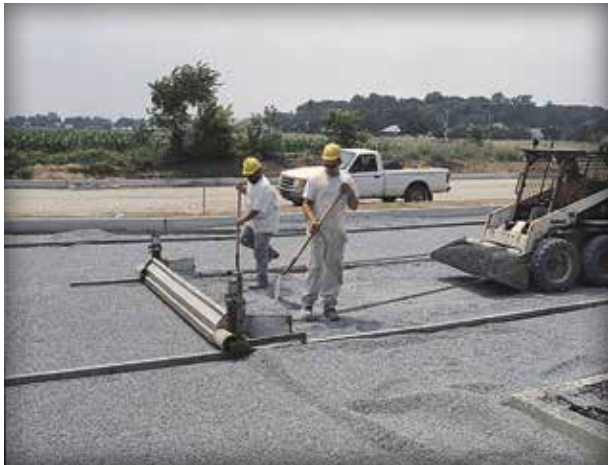
Figure 4-26. For larger areas, bucket screeds can be pulled with equipment to accelerate the screeding process.
