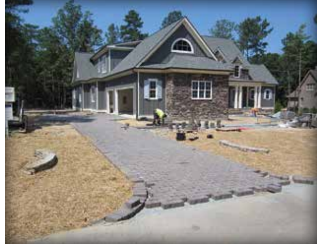
Figure 4-21. An aluminum edge restraint with geogrid is used on this residential driveway.
