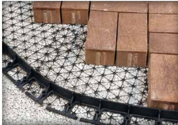
Figure 4-22. Geogrid is welded to the bottom of this plastic edge restraint.
