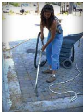
Figure 5-16. Wet/dry shop vacuum cleans loose sediment from a PICP residential driveway
