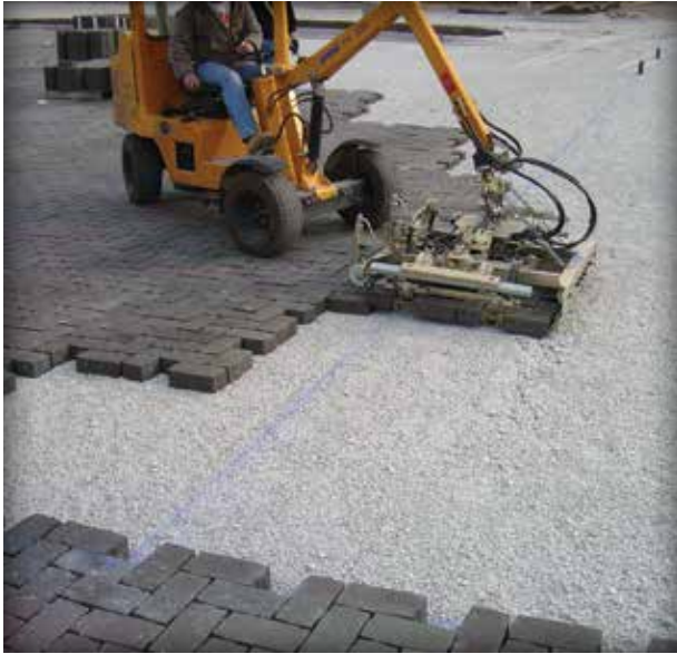
Figure 4-28 and 4-29. Mechanical equipment accelerated installation of a parking lot in Illinois and a street in Oregon.
