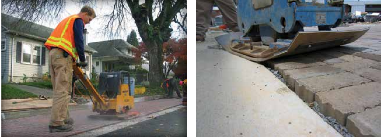
Figure 4-31. Prior to compaction, concrete pavers are typically as set about 1 in. (25 mm) higher than adjacent surfaces or curbs. The right-hand picture shows a pad under the plate compactor to protect the pavers' surfaces from scratches during compaction.
