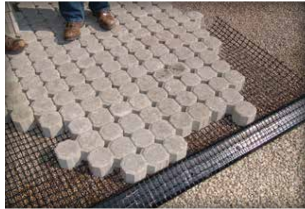
Figure 4-23. Geogrid is wrapped around this plastic edge restraint.
