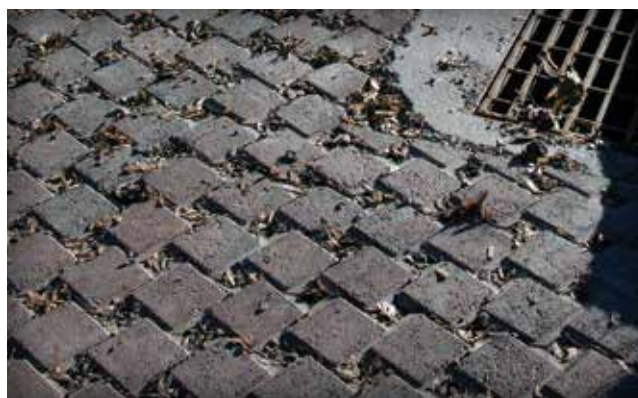
Figures 5-6 and 5-7. Pine needles and leaves eventually will degrade and get compacted into the joints from traffic. They should be removed by sweeping or vacuuming before that happens.
