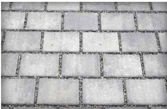
Figure 5-3. Keeping PICP joints filled with permeable aggregate facilitates removal of accumulated sediment.
