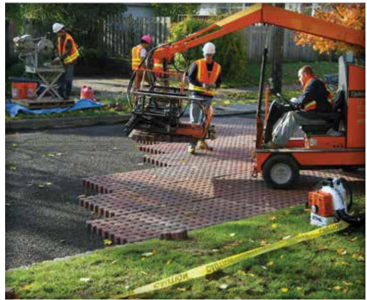
Figure 4-28 and 4-29. Mechanical equipment accelerated installation of a parking lot in Illinois and a street in Oregon.
