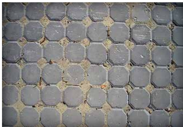
Figure 5-5. Sand from winter maintenance must be removed the following spring.
