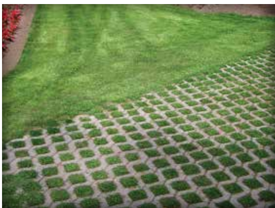
Figure 1-4. Concrete grid pavements are a permeable pavement but are used in intermittently trafficked areas.
