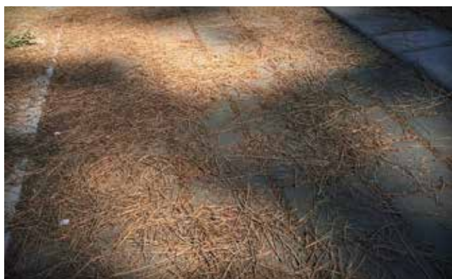
Figures 5-6 and 5-7. Pine needles and leaves eventually will degrade and get compacted into the joints from traffic. They should be removed by sweeping or vacuuming before that happens.
