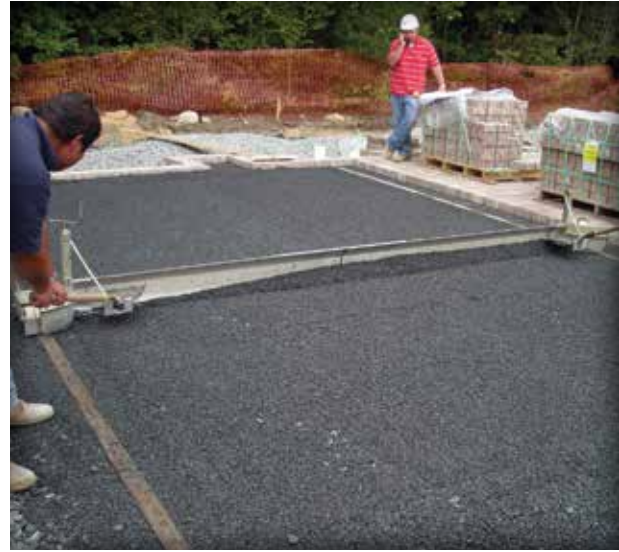
Figure 4-25. A bucket screed powered manually is used to screed parking spaces.
