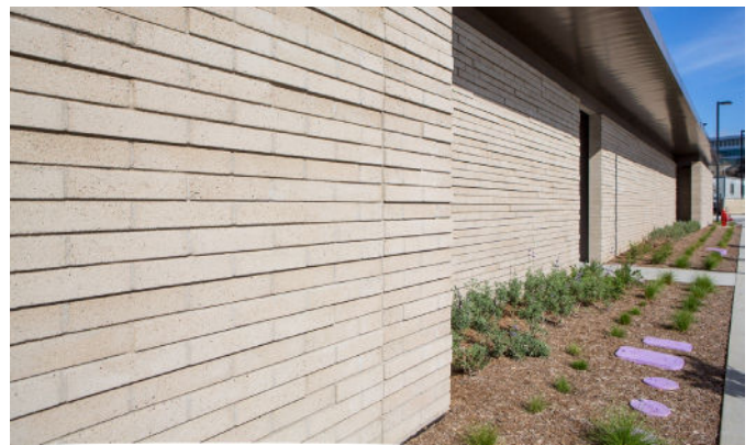
FIGURE 17—Sandblasted Units
