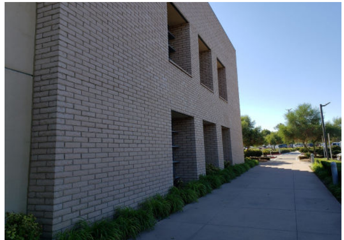
FIGURE 20—Slump Block Units
