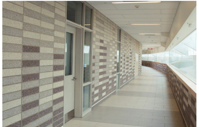
FIGURE 16—Ground Faced Units
