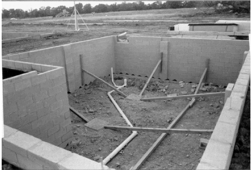
Figure 8-6: Bracing of Masonry Foundation
