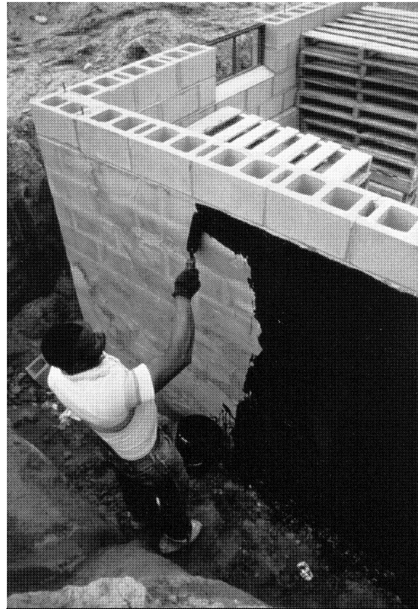
Figure 4-10: Applying Exterior Bituminous Sealant
