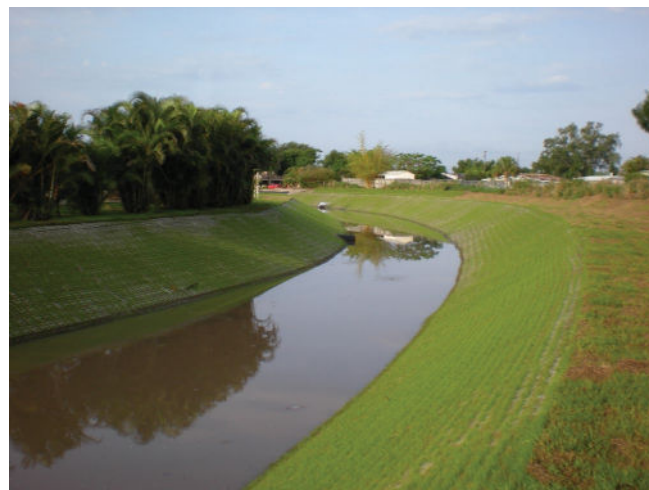
Stream Channelization, Before and After ACB Installation
