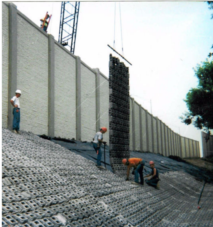
Figure 6—Cabled ACB Installation Behind a Sound Barrier
