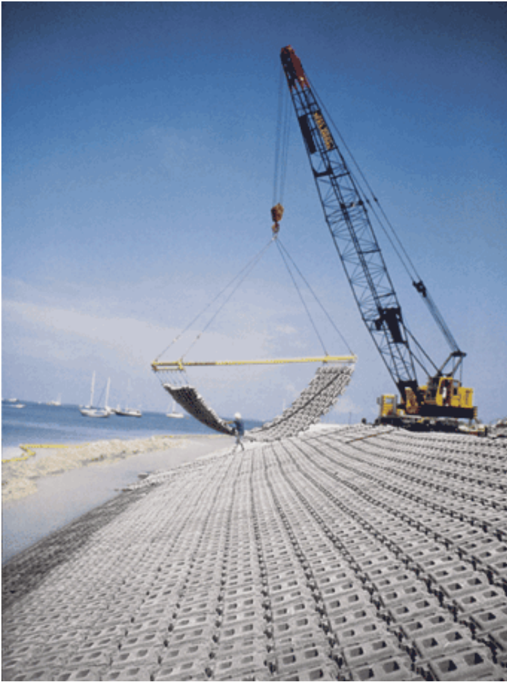
Figure 5—Placement of Cable ACB System With Crane
