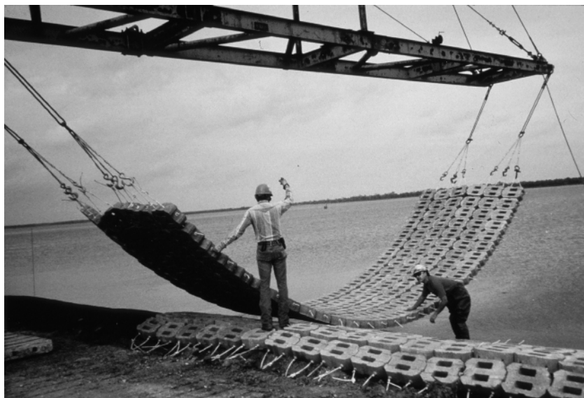
Figure 7.3—Close-up of spreader bar and ACB mat.
