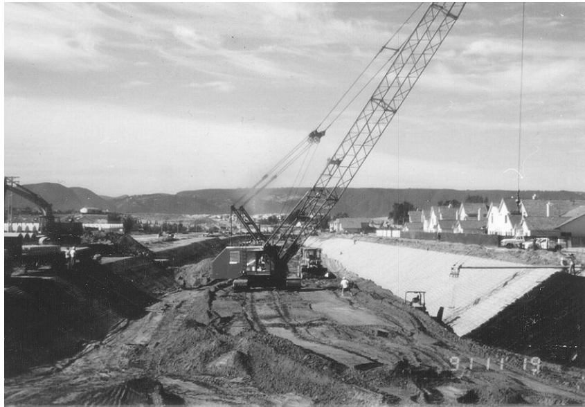
Figure 7.2—ACB mats being placed with a crane and spreader bar.
